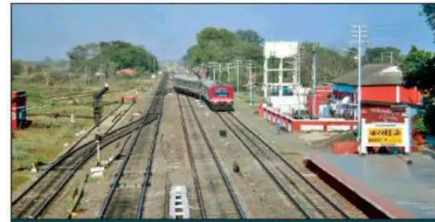
A train enters a loop line to reach a platform
